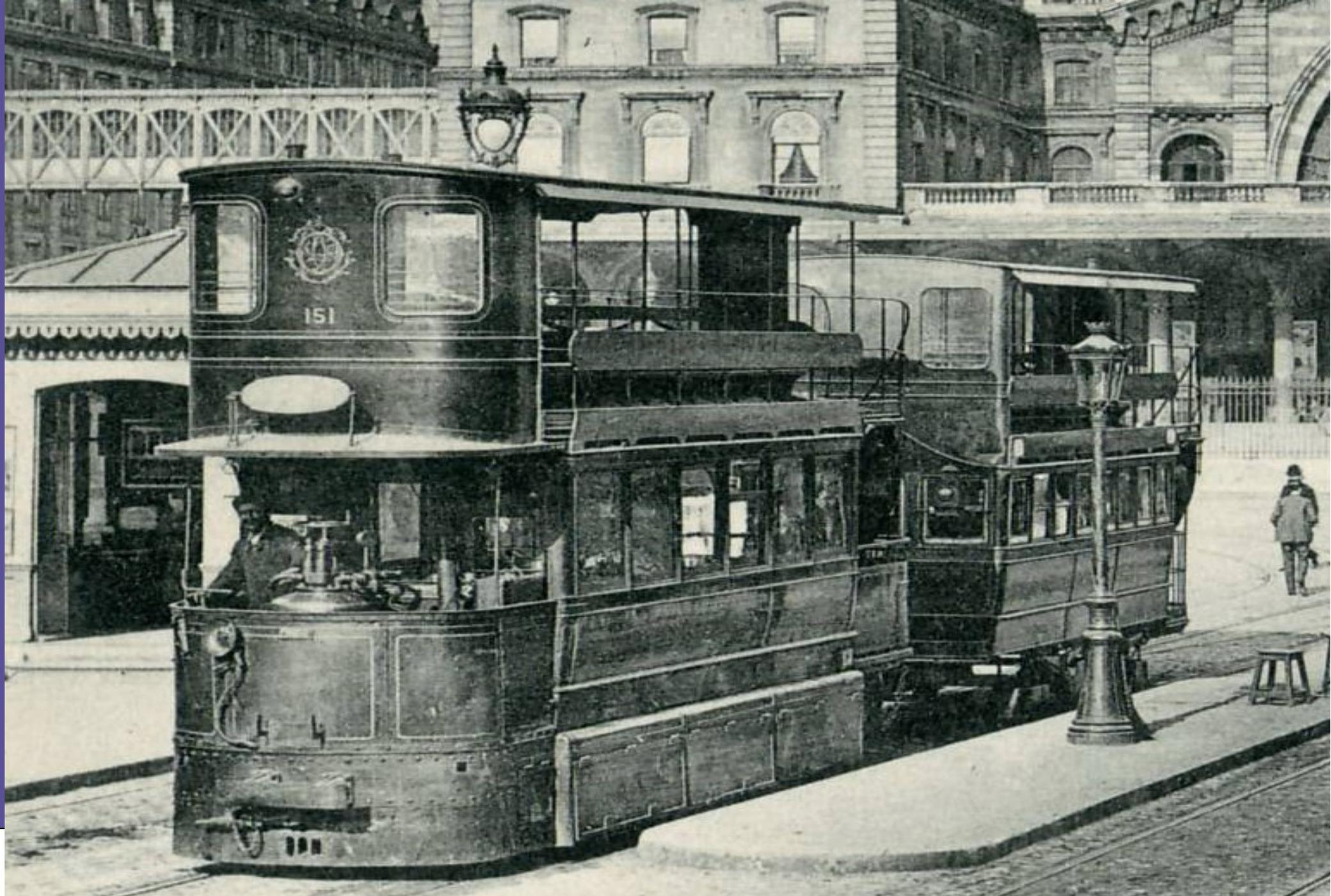
**Tramway with pneumatic engine in Paris (1900)**
